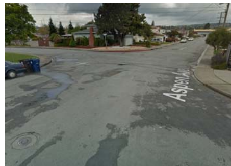
Intersection of Aspen Avenue and Pine Street looking West along Pine Street
