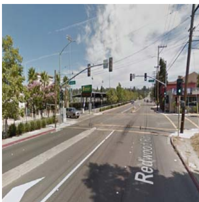
Redwood Road at Heyer Avenue looking North
